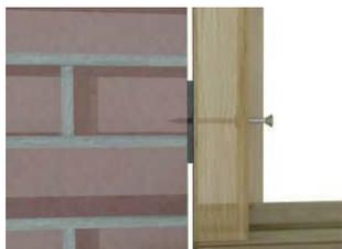
You can fix into the brickwork using either a screw and anchor plug or self tapping concrete anchor, ensure the fixing is at least 25mm into the brickwork, preferably 50mm. We recommend using an 8x120mm fixing (can be purchased from our website). Both the frame and brickwork will need to be drilled creating a pilot hole to fix into.
